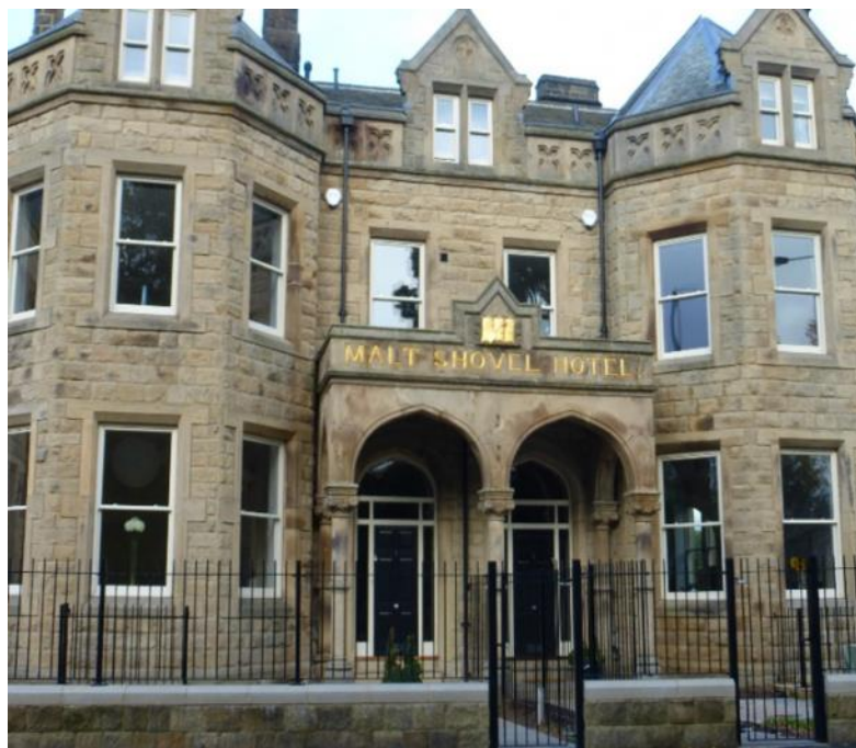
The Malt Shovel an example of a former hotel within Burley adapted for new residential use.
